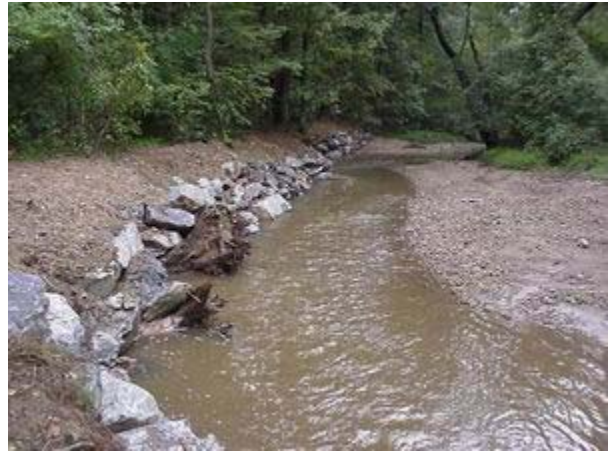
PAINT BRANCH - AFTER STREAM RESTORATION
