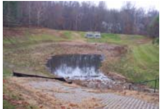
SNOWDENS MILL II STORMWATER MANAGEMENT RETROFIT (MONTGOMERY COUNTY)
