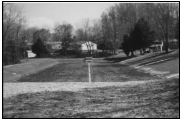
Figure 17. Hollywood Branch Peat Sand Filter, Montgomery County.
