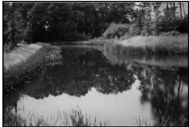
Figure 18. Kentlands No. 2 Wetland, Prince George's County.
