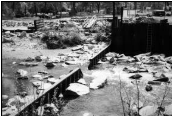
Figure 29. Northeast Branch Weir Fish Barrier Modification Work, 1991.
