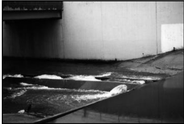
Figure 31. Northwest Branch U.S. Army Corps of Engineers Denil Fish Ladder at U.S. Route 1, 1995.
