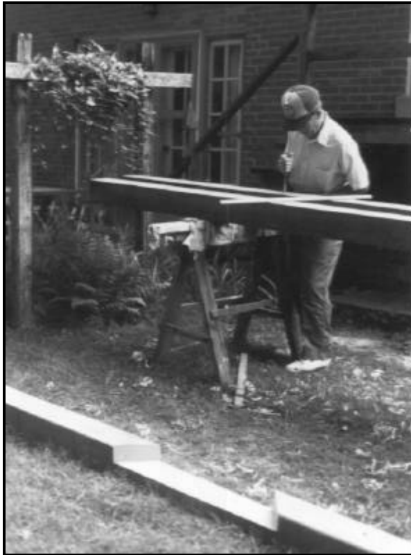
Figure 45. Trout Unlimited Construction of Gum Springs Check Dams, 1990.
