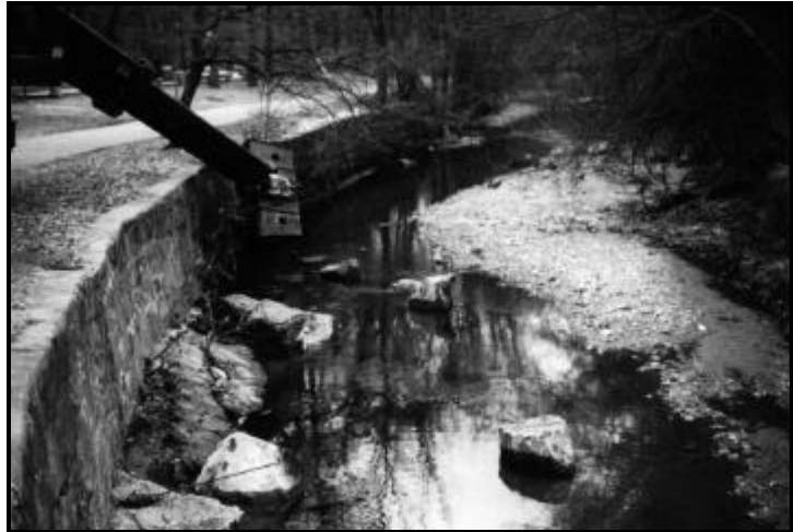
Figure 23. Boulder Placement: Sligo Creek Stream Restoration Phase II, 1994.
