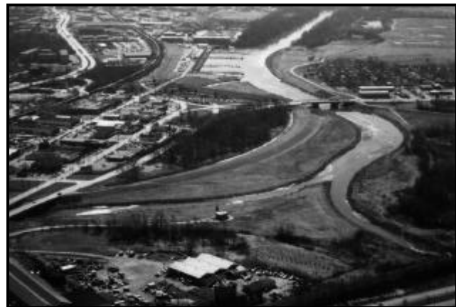
Figure 35. Northeast and Northwest Branches Confluence (foreground) with the Anacostia River.
