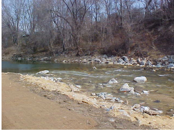
Figure 5. Stream restoration on Northwest Branch at NW2
