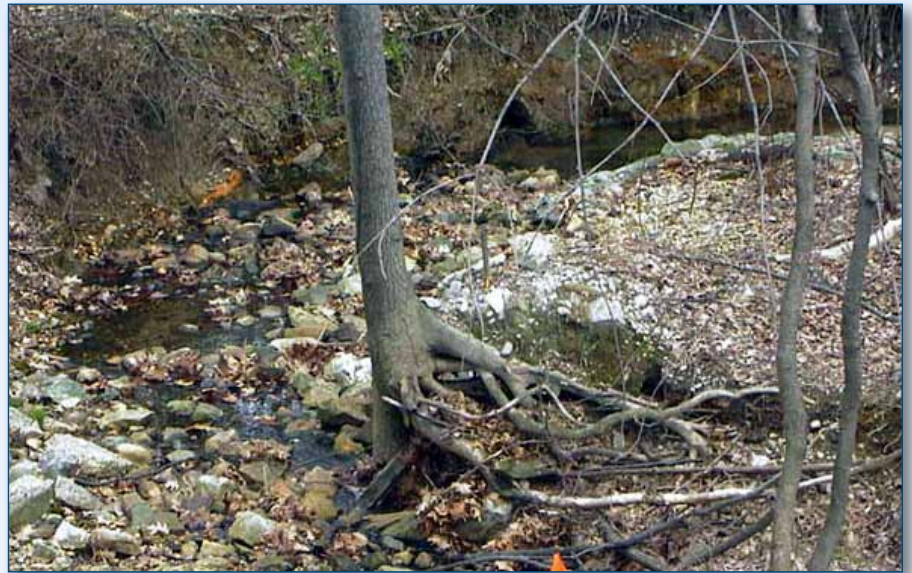
Figure 1-2: Channel entrenchment and streambank erosion
