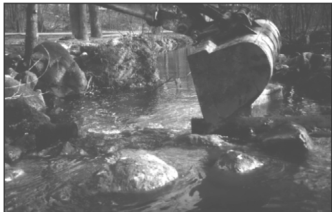
Sligo Creek Phase IV Restoration.
