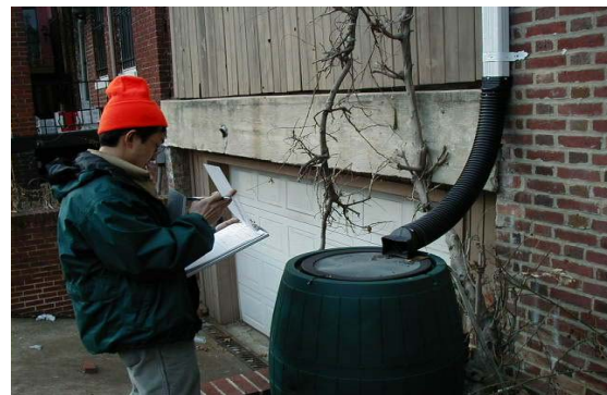
Figure 13. Rain Barrel Inspection by COG Staff
