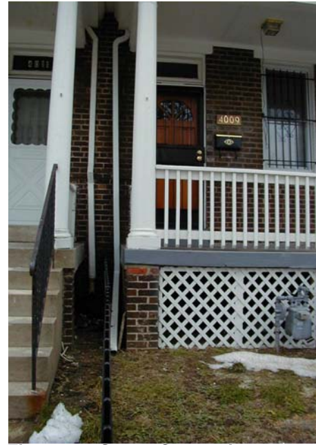
Figure 11. Space Constraints around Row Houses Limit Barrel Placement
