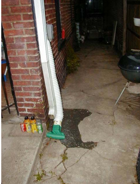
Figure 9. Rain Barrel Site No. 8 Prior to Installation
