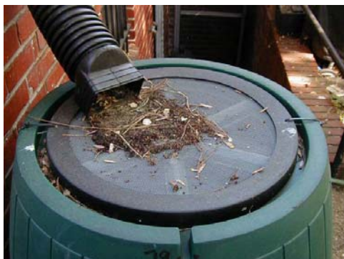
Figure 14. Organic Debris on Rain Barrel Screen
