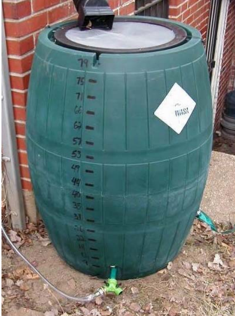
Figure 7. Barrel with Water Level Indicator Hose and Gallon Marks
