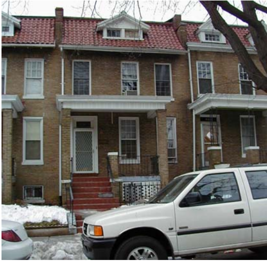
Figure 5. Typical Washington DC Rowhouse
