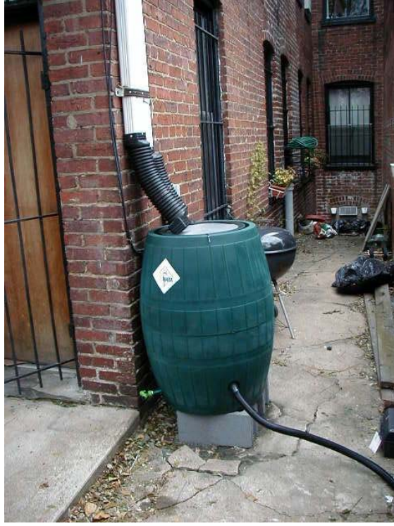
Figure 10. Site No. 8 Site After Rain Barrel Installation
