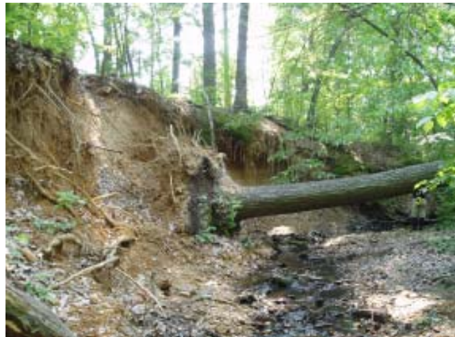
Figure 5 - Upper reach - Severe Streambank Erosion
