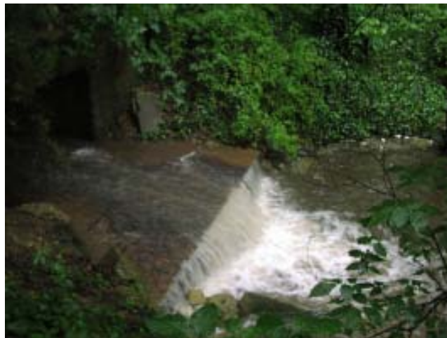
Figure 29 - Upper Reach - Texas Avenue Storm Drain Outfall (4'Hx8'W) Uncontrolled Runoff During a July 11, 2003 Afternoon Thunderstorm
