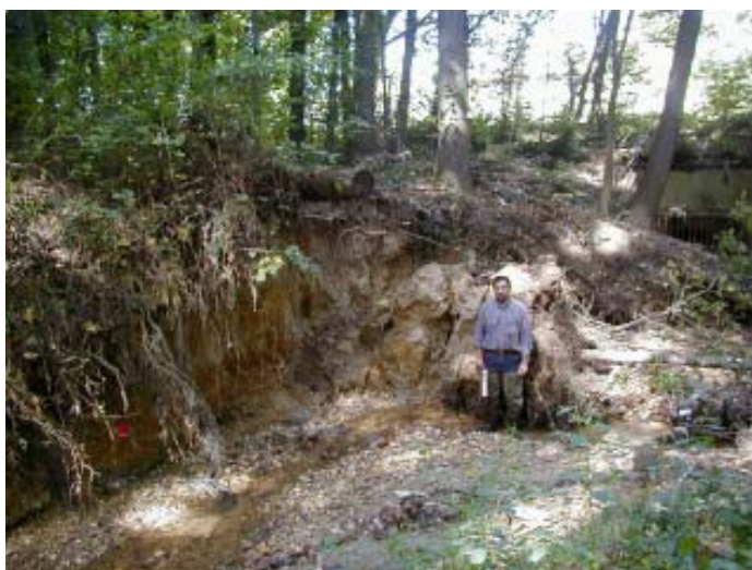
Figure 7 - Lower Reach ('C' Street Area) - Severe Channel Erosion
