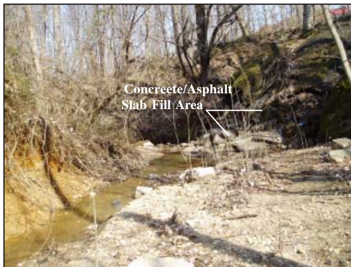
Figure 32 - Upper Reach - Right Bank Slope Failure Area
