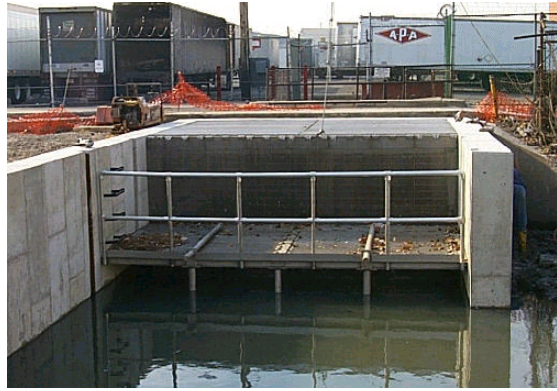
Figure 6. End-of-Pipe Fresh Creek Netting System
