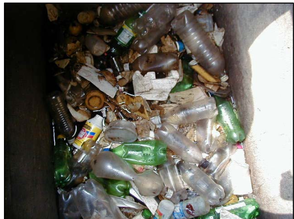
Figure 2. Anacostia CSO 018 Sewershed Storm Drain Inlet Filled with Trash and Debris
