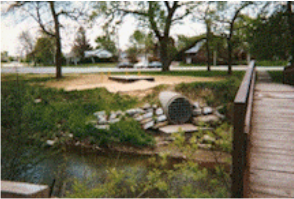
Figure 5. In-Line Fresh Creek Netting System
