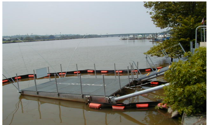
Figure 7. Floating Fresh Creek Netting System at CSO 018
