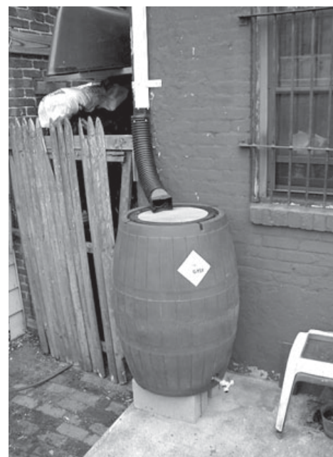
DC-WASA AND COG INSTALLED RAIN BARRELS LIKE THIS ONE AT A NUMBER OF RESIDENCES IN THE CSO PORTION OF THE WATERSHED
