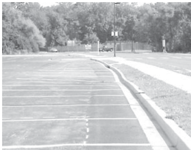
A PLANNED LID PROJECT WILL REDUCE ENVIRONMENTAL IMPACTS FROM THIS UNIVERSITY OF MARYLAND PARKING AREA
