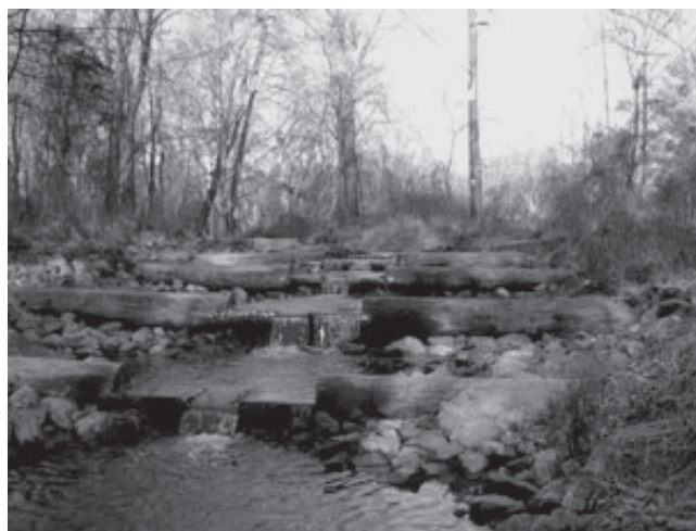
A COMPLETED PAINT BRANCH FISH PASSAGE PROJECT AT MAYDALE NATURE CENTER
