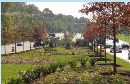
Prince George's County Green Highway
